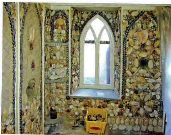
Restoration work underway
